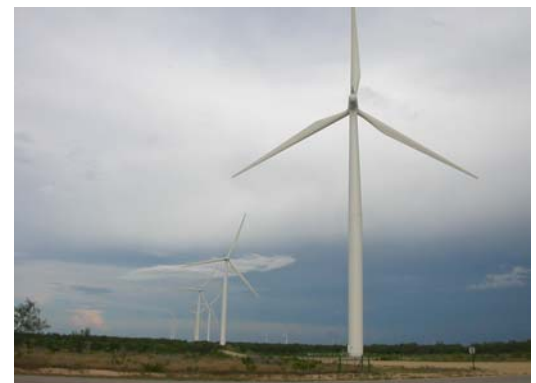
Siemens 2.3 MW generators tower above ranchland near Highland in Phase 4 of Babcock & Brown's Sweetwater project — second largest in the USA.
